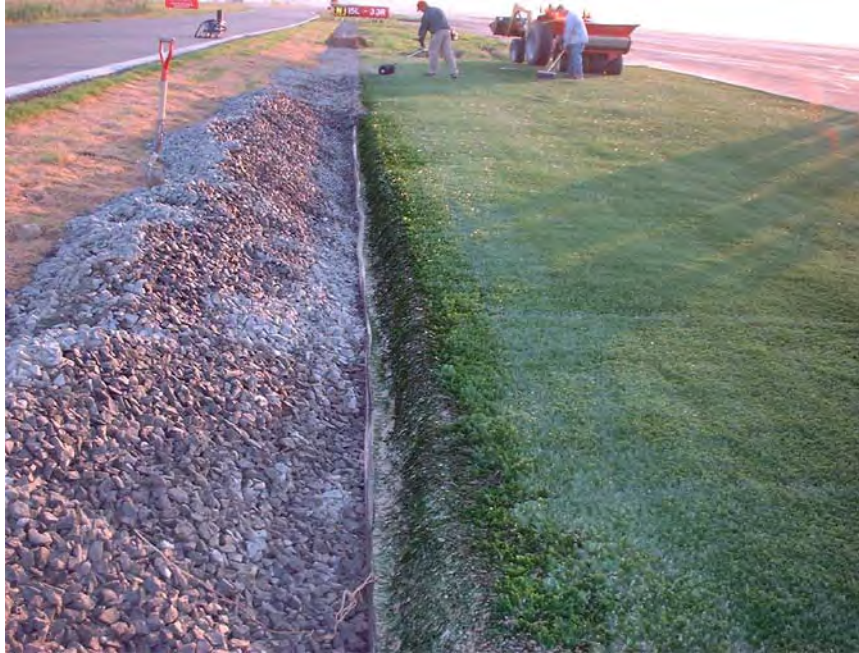
FIGURE 3-5. ARTIFICIAL TURF BACKSIDE TRENCHING AND ATTACHMENT
