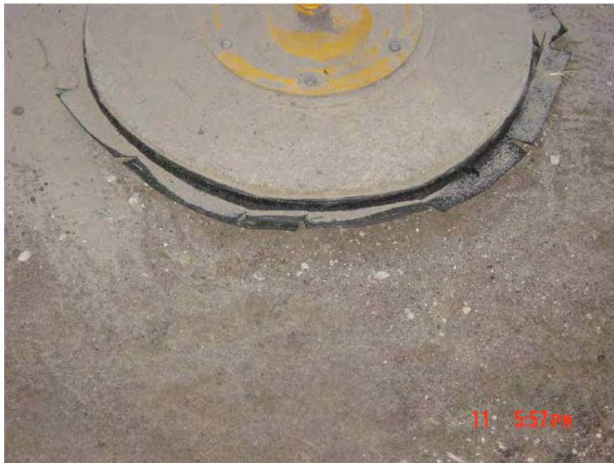
FIGURE 3-16. LIGHT CAN WITH FLEXIBLE L ANGLE INSTALLED
