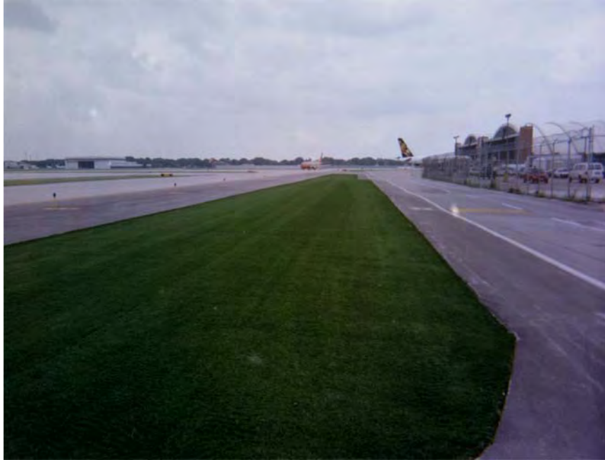
FIGURE 2-27. VISUAL ENHANCEMENT AT MDW
