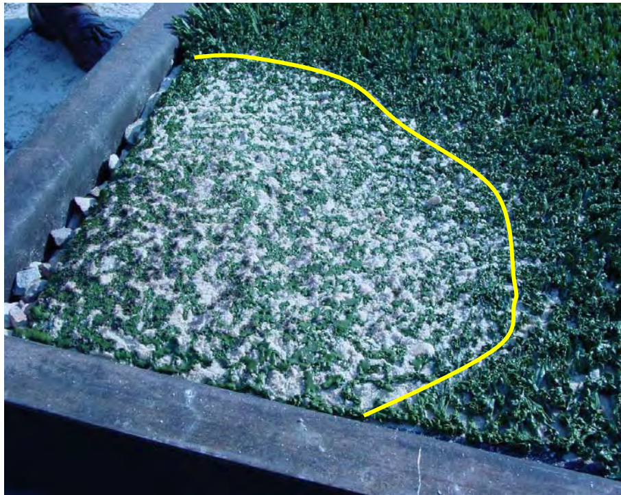
FIGURE D-15. BURNT AREA (OUTLINED IN YELLOW) FROM PROPANE TORCH
