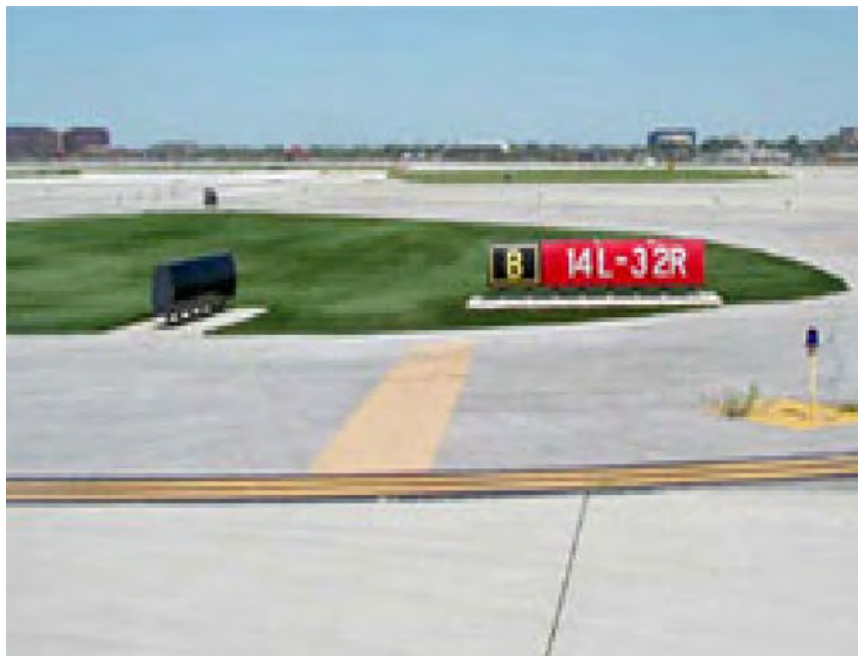
FIGURE 2-5. ARTIFICIAL TURF INSTALLATION AT ORD RUNWAY 14L/32R
