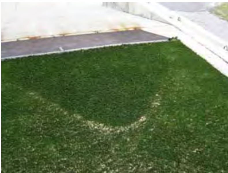
FIGURE C-14. CONE SHAPE FROM MIGRATION OF SAND
