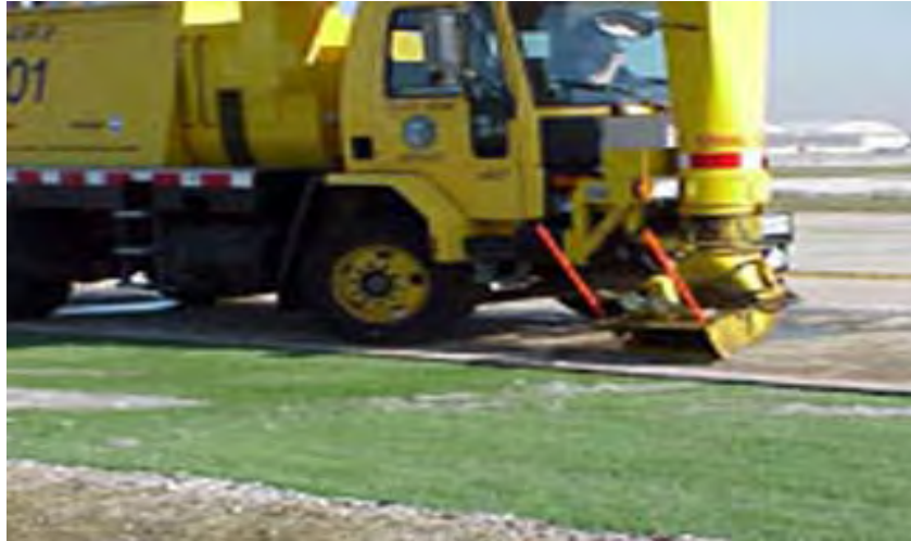
FIGURE 4-20. CONCENTRATED AIR BLOWER USED ON EDGE ATTACHMENT OF ARTIFICIAL TURF (BOS)
