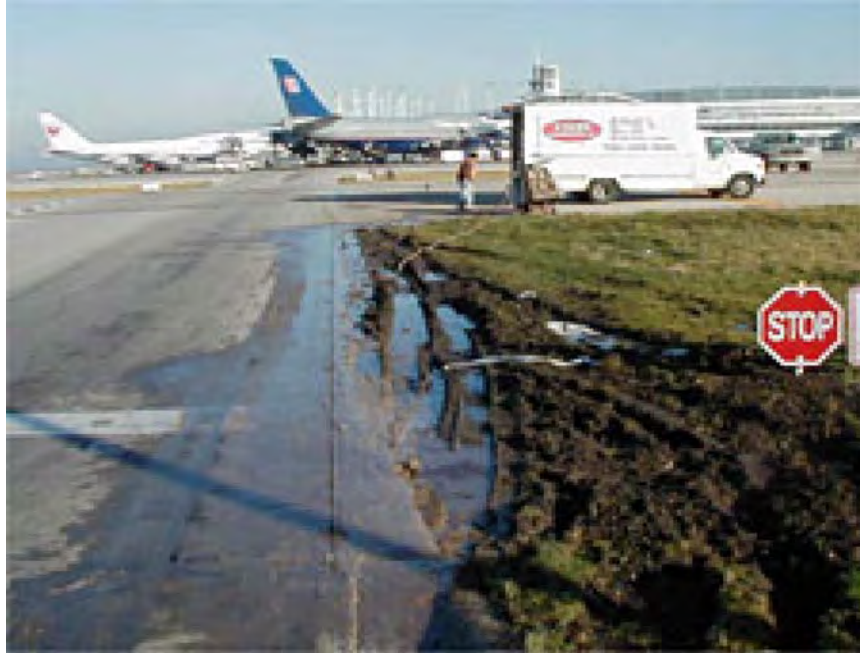
FIGURE 2-2. PROBLEM AREA AT TAXIWAY D2 (ORD) VIEW 2
