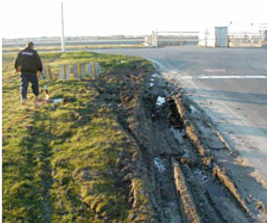
FIGURE 2-1. PROBLEM AREA AT TAXIWAY D2 (ORD) VIEW 1
