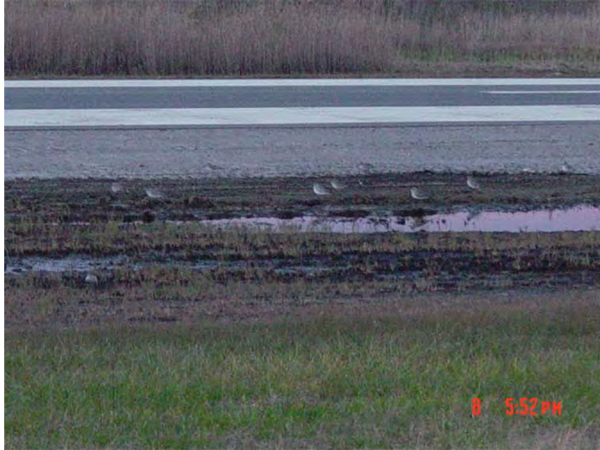
FIGURE 2-11. PONDING WATER ALONG THE EDGE OF RUNWAY 6/24 ADJACENT TO ARTIFICIAL TURF INSTALLATION LOCATION
