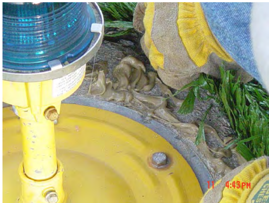
FIGURE 3-25. ARTIFICIAL TURF BEING ATTACHED TO A LIGHT-MOUNTING FIXTURE
