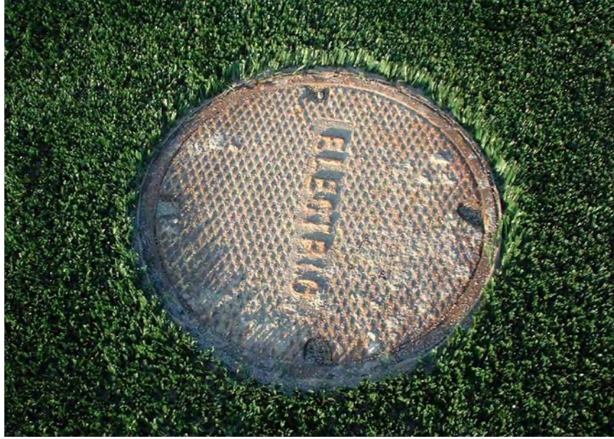
FIGURE 3-7. ARTIFICIAL TURF INSTALLED AROUND EXISTING MANHOLE COVER
