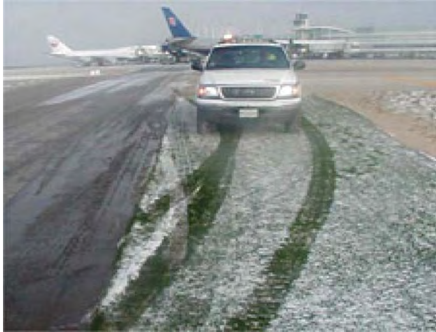
FIGURE 2-4. ARTIFICIAL TURF AT ORD TAXIWAY D2
