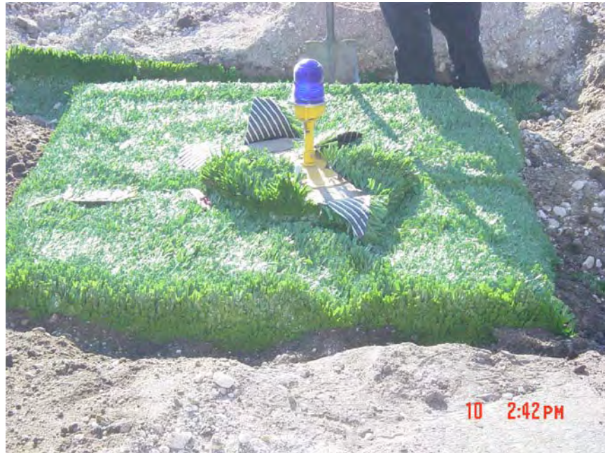
FIGURE 3-23. TRENCHED ARTIFICIAL TURF PLACED AROUND LIGHT CAN
