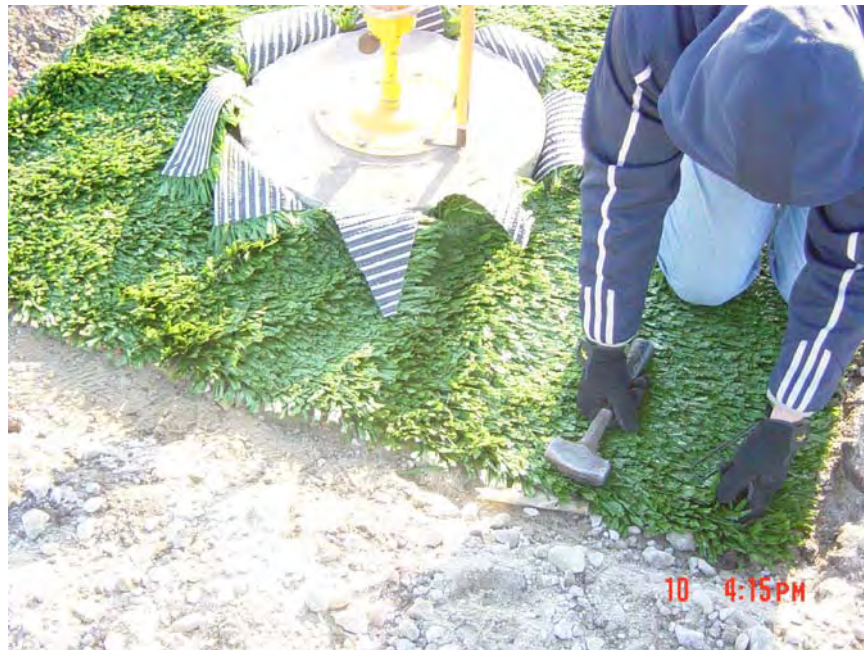
FIGURE 3-18. TURF-PEGGING ARTIFICIAL TURF TO GROUND
