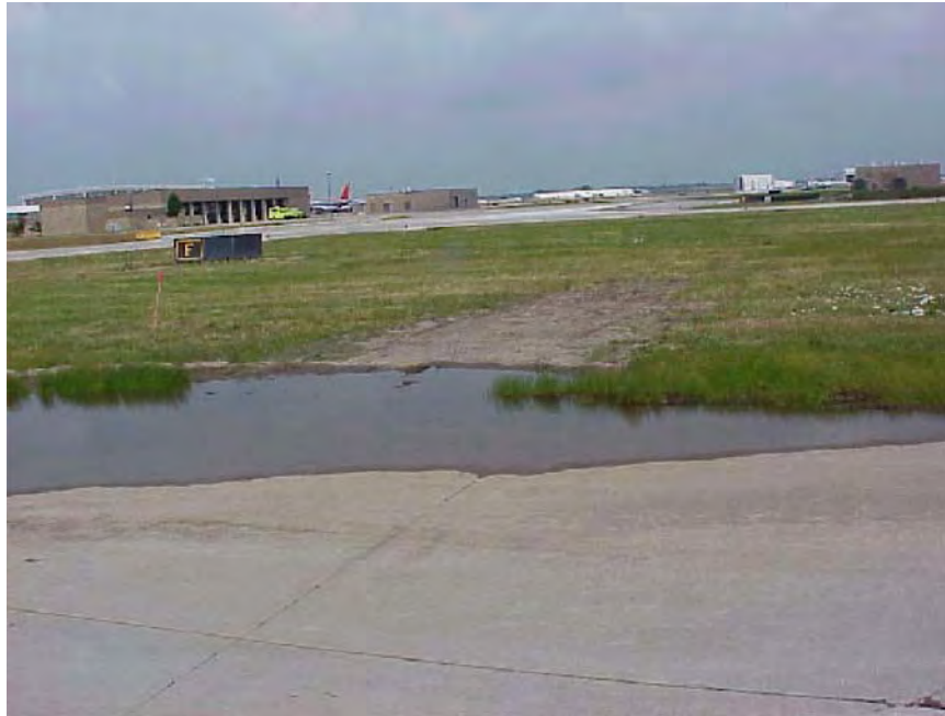
FIGURE 2-24. TEST LOCATION AT DTW RUNWAY 4R/22L, PREINSTALLATION
