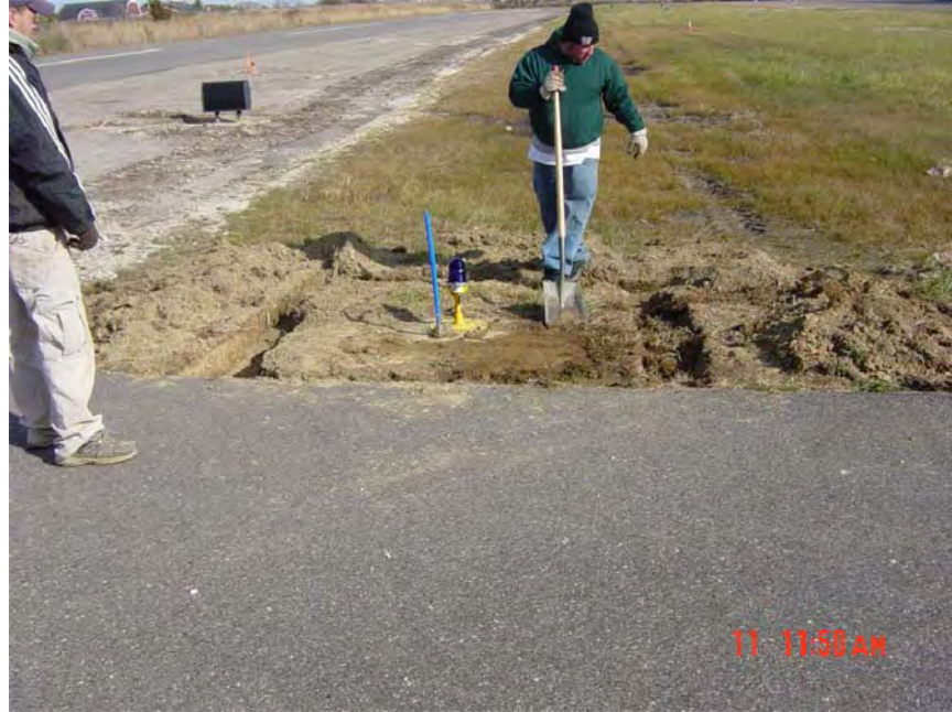
FIGURE 3-22. LIGHT CAN BEING TRENCHED FOR INSTALLATION OF ARTIFICIAL TURF
