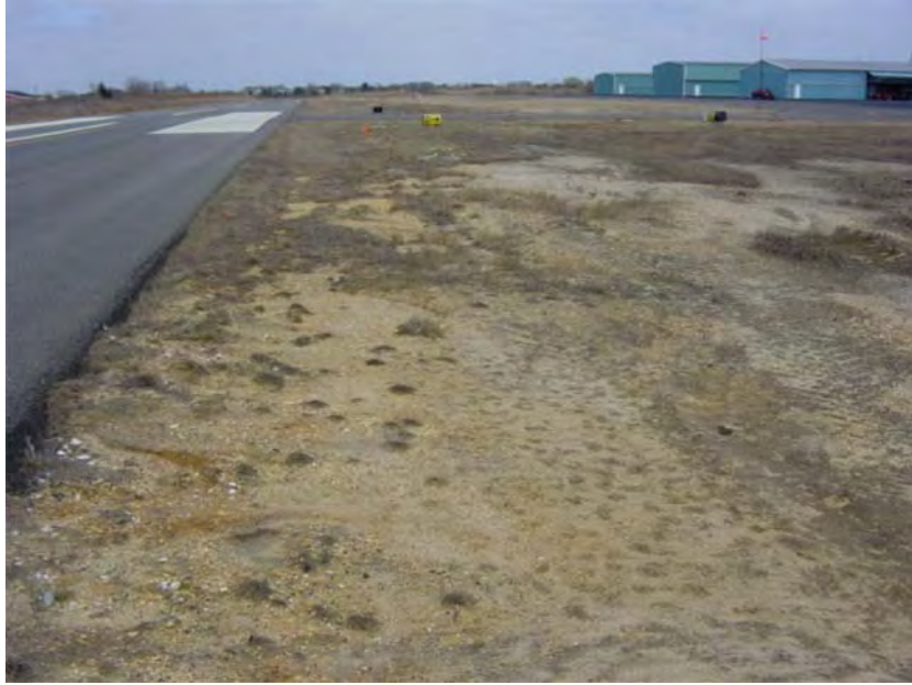
FIGURE 2-9. TEST PLOT LOCATION PRIOR TO ARTIFICIAL TURF INSTALLATION ON RUNWAY 6/24 (SOIL EROSION)
