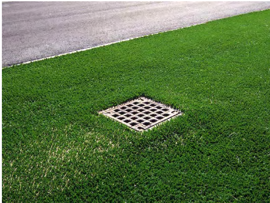
FIGURE 3-8. ARTIFICIAL TURF INSTALLED AROUND EXISTING ACCESS DRAIN
