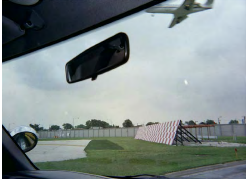
FIGURE 4-22. ARTIFICIAL TURF INSTALLED AT MDW BLAST PAD LOCATION
