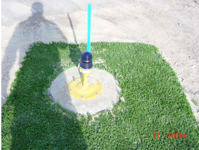
FIGURE 3-19. COMPLETED INSTALLATION AROUND LIGHT CAN
