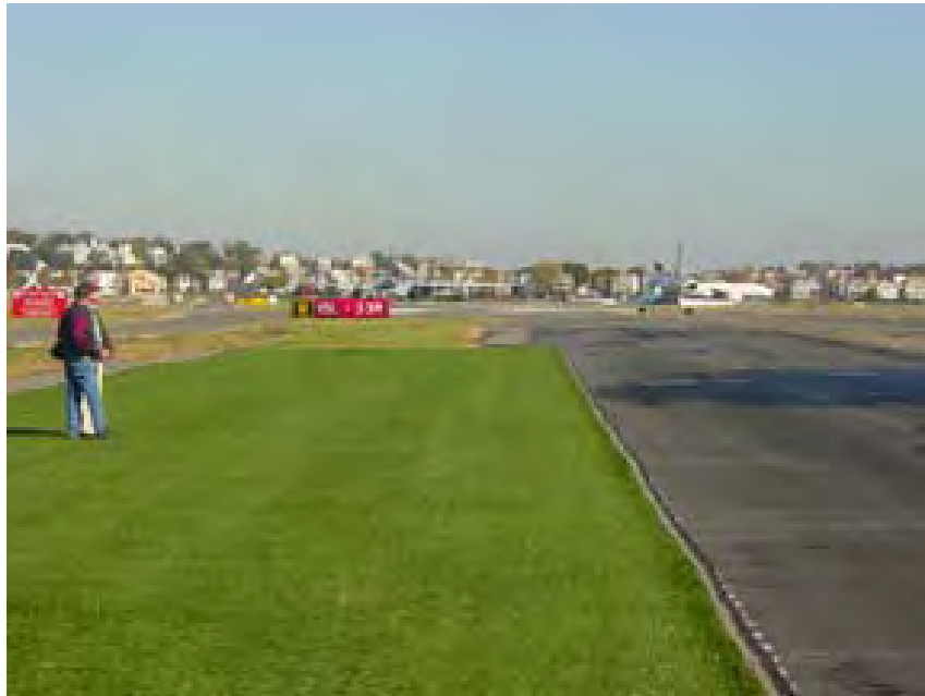
FIGURE 2-8. TEST LOCATION AT BOS TAXIWAY N, POSTINSTALLATION
