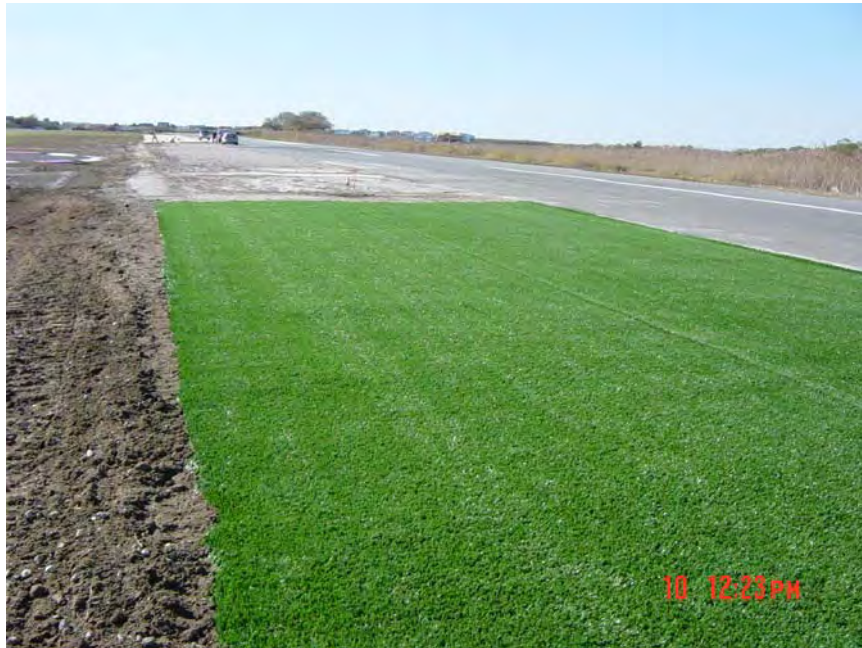
FIGURE 2-12. ARTIFICIAL TURF INSTALLATION ALONG THE EDGE OF RUNWAY 6/24 VIEW 1
