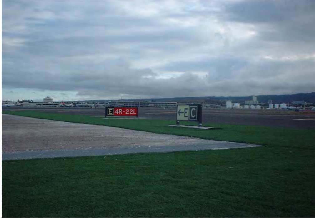
FIGURE 2-15. SITE VIEW WITH ARTIFICIAL TURF INSTALLED (HNL)
