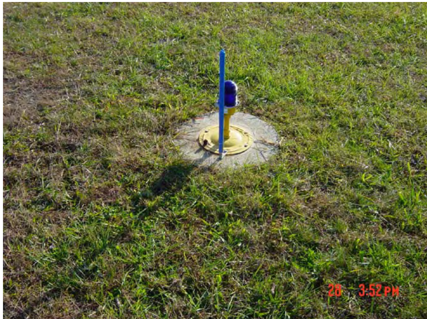
FIGURE 3-14. LIGHT CAN PRIOR TO ARTIFICIAL TURF BOX INSTALLATION
