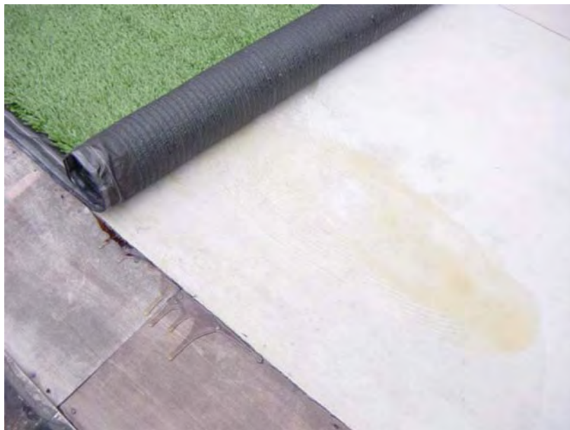
FIGURE 3-13. APPLICATION OF NORDOT 34N ON CONCRETE
