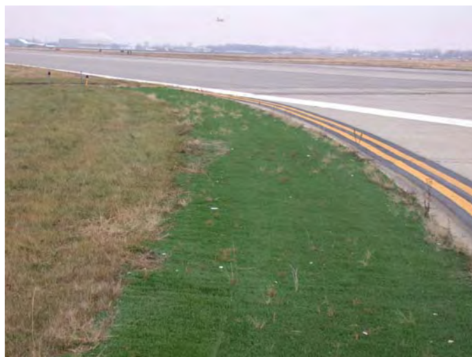
FIGURE 2-19. TEST LOCATION AT DTW RUNWAY 4R/22L, POSTINSTALLATION
