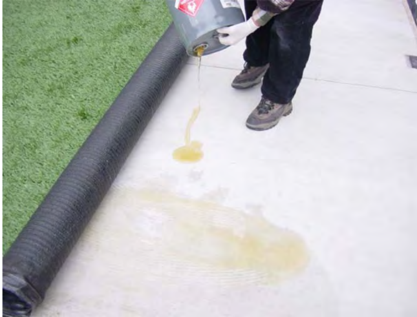
FIGURE C-39. APPLICATION OF ARTIFICIAL TURF TO CONCRETE
