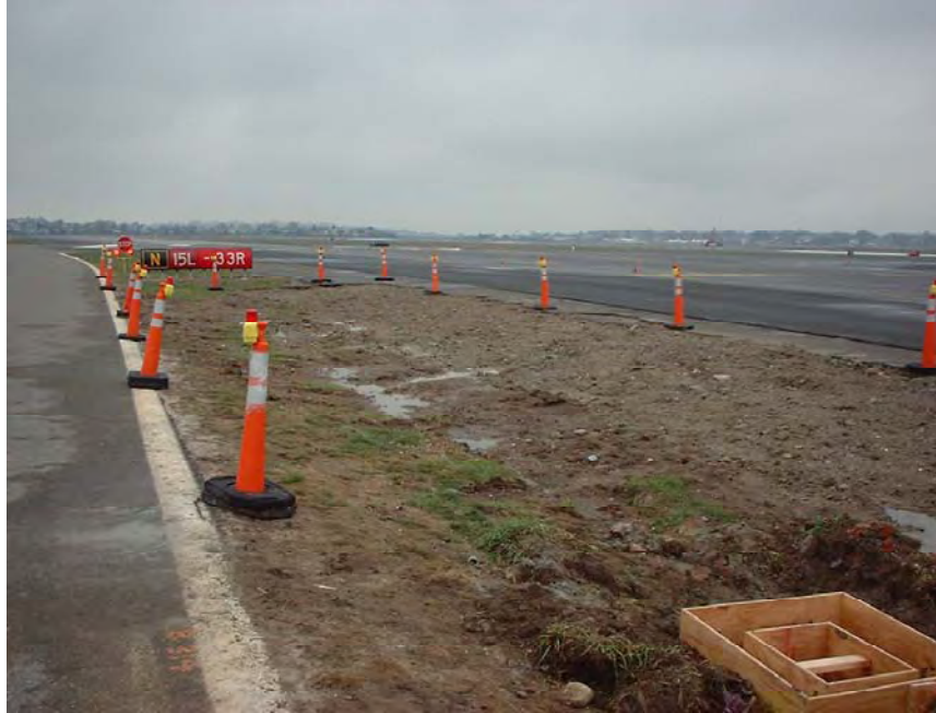
FIGURE 2-7. TEST LOCATION AT BOS TAXIWAY N, PREINSTALLATION
