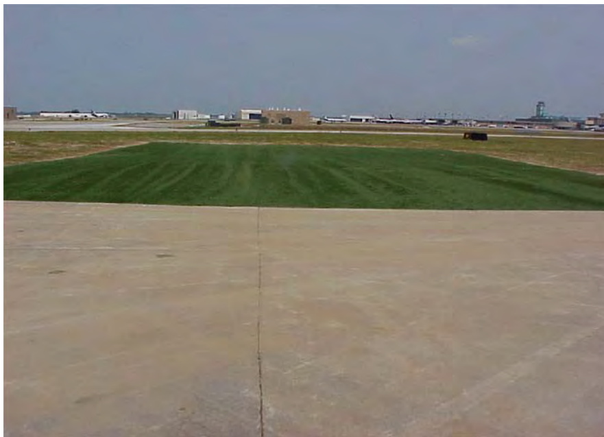
FIGURE 2-25. TEST LOCATION AT DTW RUNWAY 4R/22L, POSTINSTALLATION
