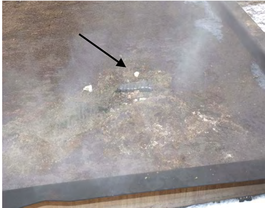
FIGURE D-13. DAMAGED BACKING MATERIAL
