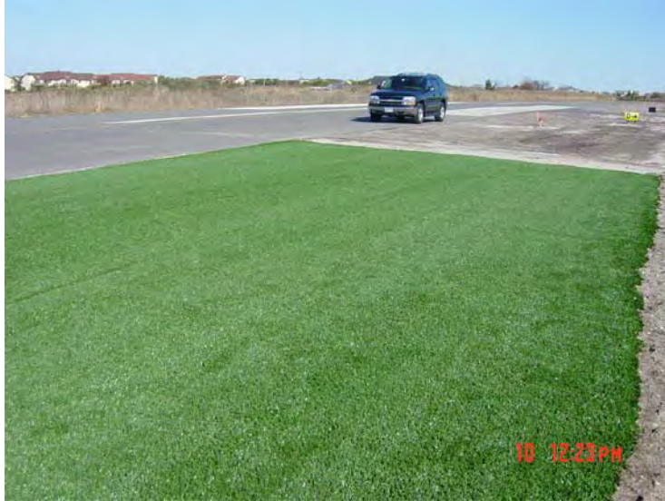
FIGURE 2-13. ARTIFICIAL TURF INSTALLATION ALONG THE EDGE OF RUNWAY 6/24 VIEW 2
