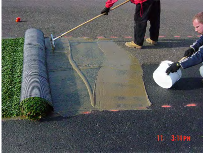
FIGURE 3-12. APPLICATION OF ENVIRONSTICK TWO-PART GLUE ON ASPHALT
