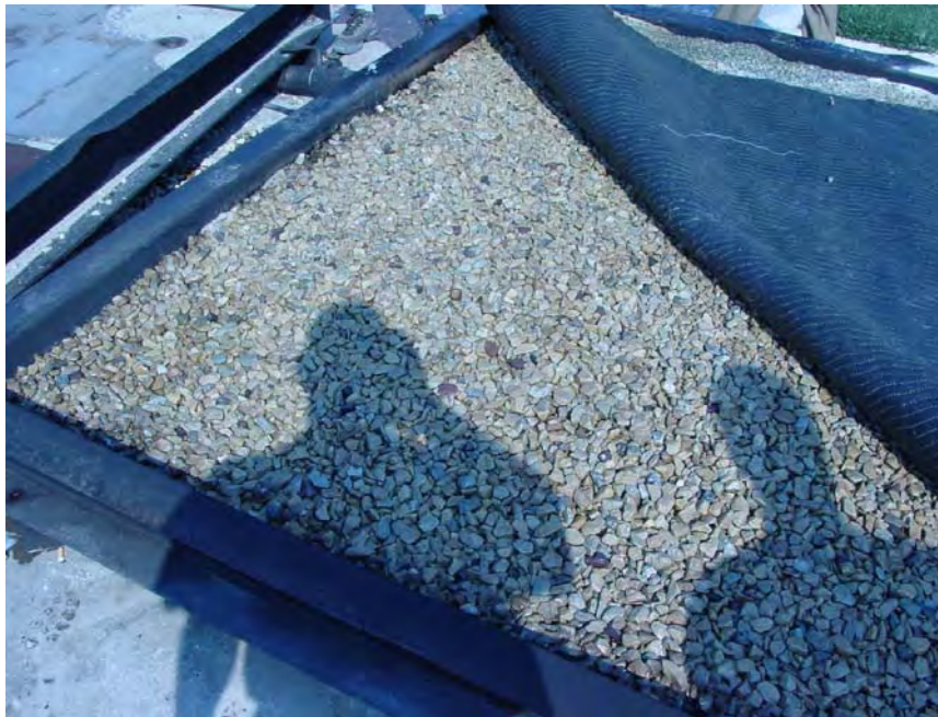
FIGURE D-21. BASE MATERIAL WITH NO FUEL CONTAMINATION
