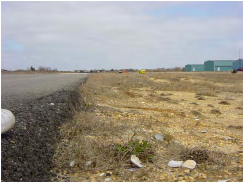
FIGURE 2-10. CLOSE-UP VIEW OF SOIL EROSION ALONG THE EDGE OF RUNWAY 6/24
