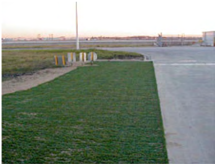
FIGURE 2-3. ARTIFICIAL TURF INSTALLED AT TAXIWAY D2 (ORD)
