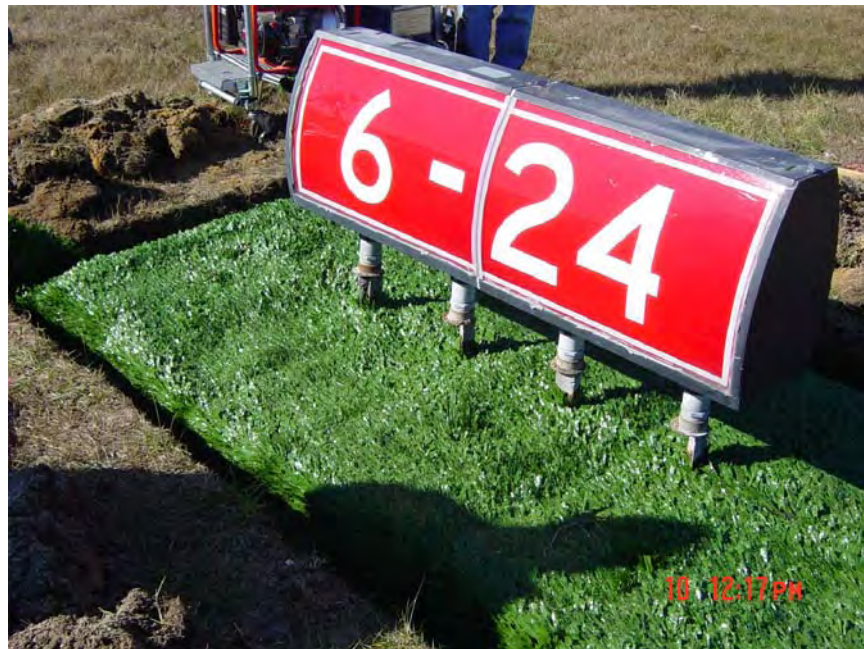
FIGURE 3-24. TRENCHED ARTIFICIAL TURF PLACED AROUND SIGN
