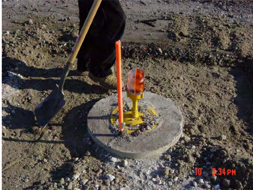
FIGURE 3-15. LIGHT CAN WITH INSTALLATION AREA DUG OUT
