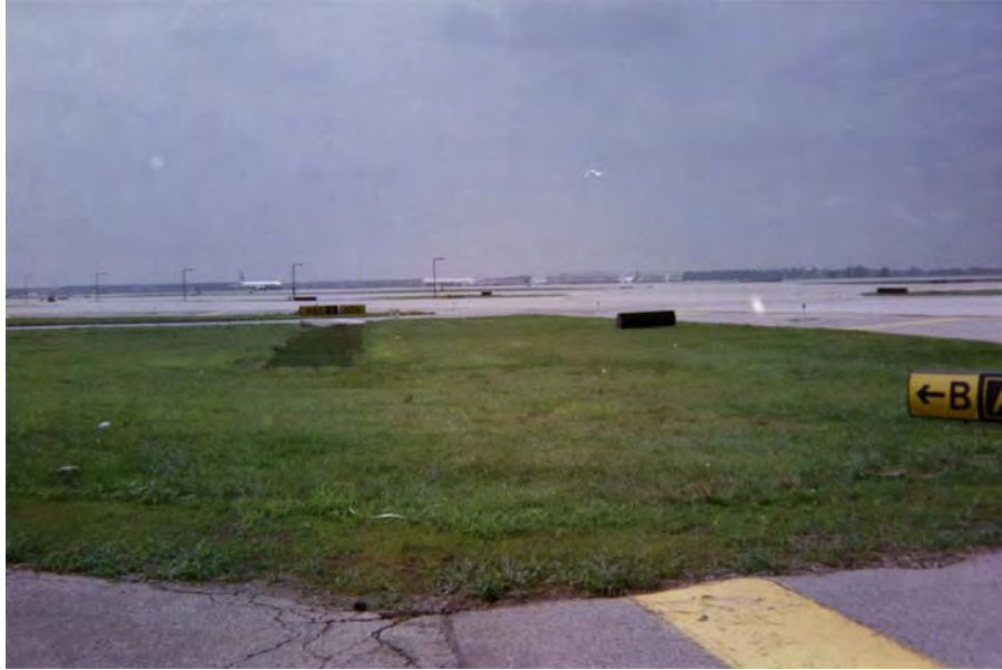
FIGURE 2-22. ARTIFICIAL TURF INSTALLATION AT ORD TAXIWAYS A6 AND A7
