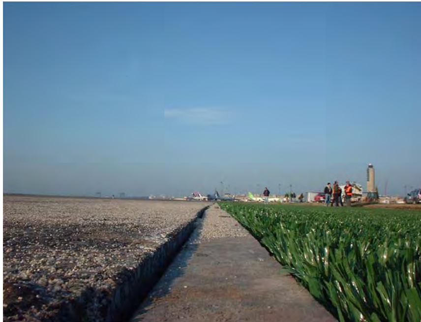
FIGURE 3-4. ARTIFICIAL TURF PAVEMENT SIDE ATTACHMENT
