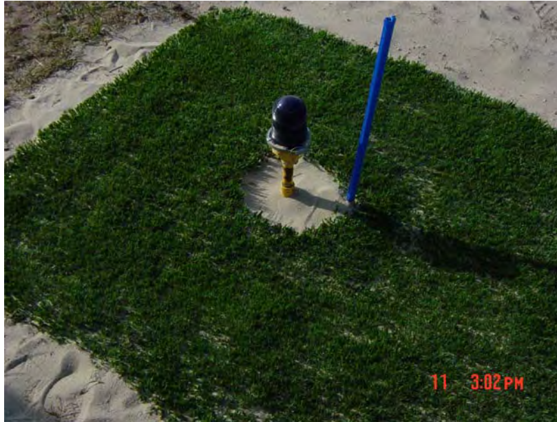
FIGURE 3-26. TRENCHED ARTIFICIAL TURF INSTALLATION AROUND THE LIGHT CAN COMPLETED
